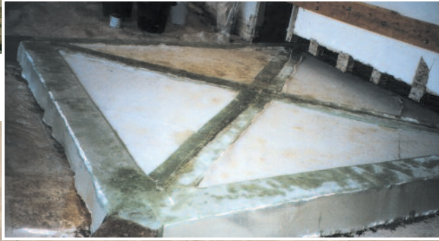
9 - Laying of last strip of woven glass fabric
