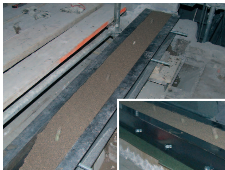
4 - Pouring the compression table using a resin mortar
