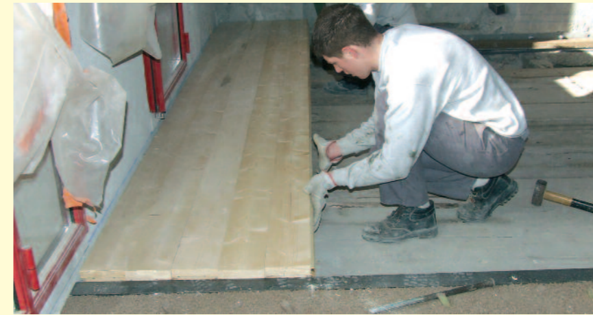
6 - Laying of first elements of the floor
