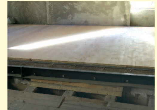
7 - Supporting ironwork awaiting laying of second part of floor
