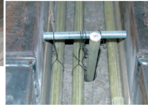
2 - Installation of glass fibre reinforcements
