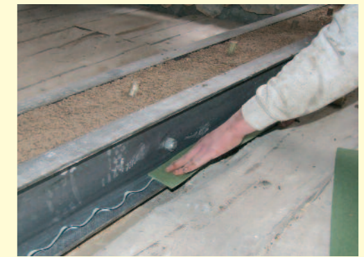
5 - Laying of soundproofing sealant
