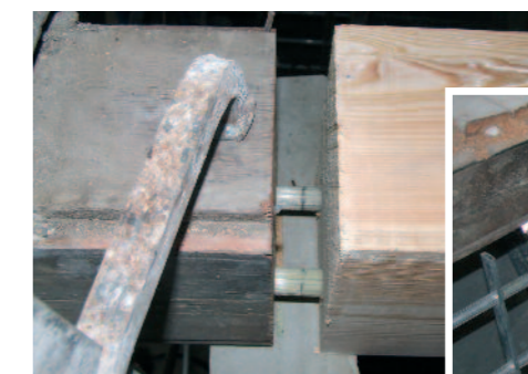
Connection of the prosthesis of a restored antique joist
